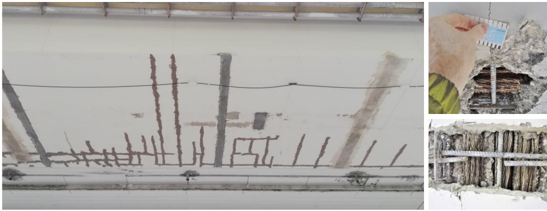
Figure 5. Visual inspection campaign carried out on the bridge.
